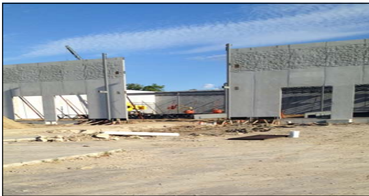
LA Fitness under construction
